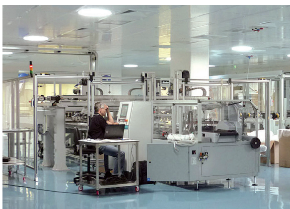
Fresenius laboratory with light pipes, Baggilux, Italy
