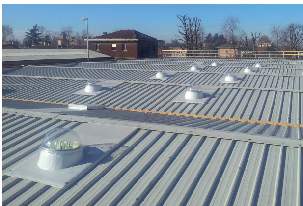
Roof at Gimec, Baggilux, Italy
